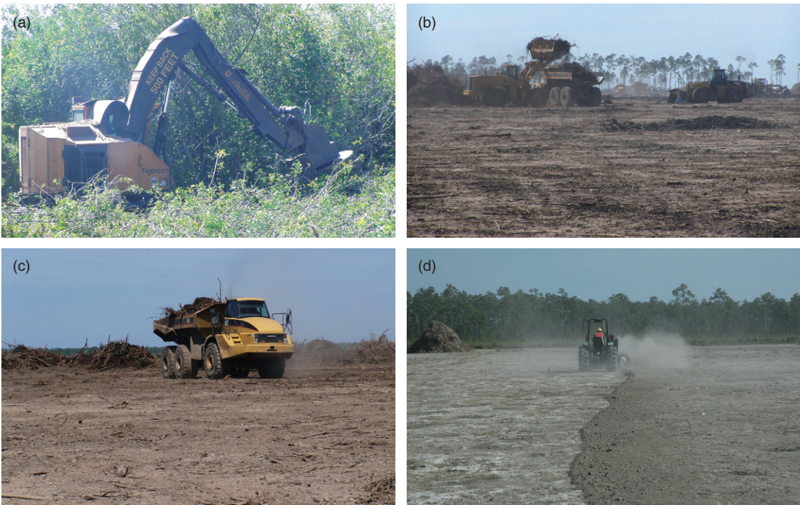
Figure 2.3 In the mid-1990s the decision was made to remove the anthrosol. The process, still underway, consists of: (a) cutting the vegetation; (b) loading the debris and soil; (c) hauling the material to local repositories within the Hole-in-the-Donut; and finally (d) scraping the remaining soil off the underlying limestone base rock. Photographs courtesy of Everglades National Park.
